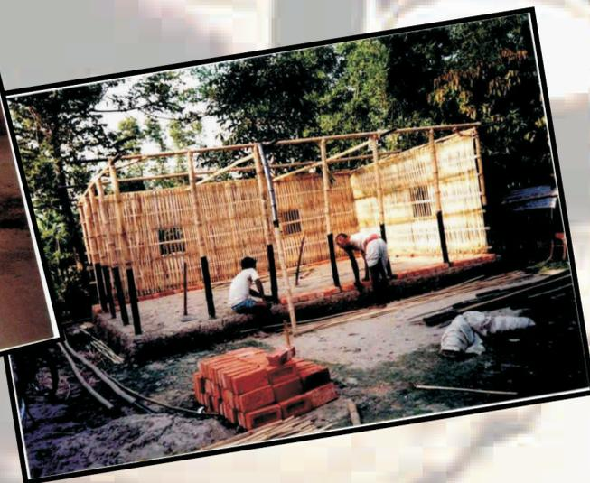
ENHANCING THE PRACTICAL USE OF NATURAL MATERIALS FOR LONG TERM AND SAFE BUILDING SOLUTIONS BY EMPLOYING TRADITIONAL METHODS FOR TREATMENT OF BAMBOO AND PROVIDING STRUCTURAL STRENGTH.....
