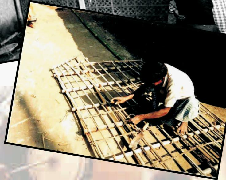
CROSS BRACING IN BAMBOO NOT ONLY PROVIDES STRUCTURAL STABILITY AND WIND RESISTANCE BUT CAN BE EXPLOITED FOR AESTHETICS TOO....
